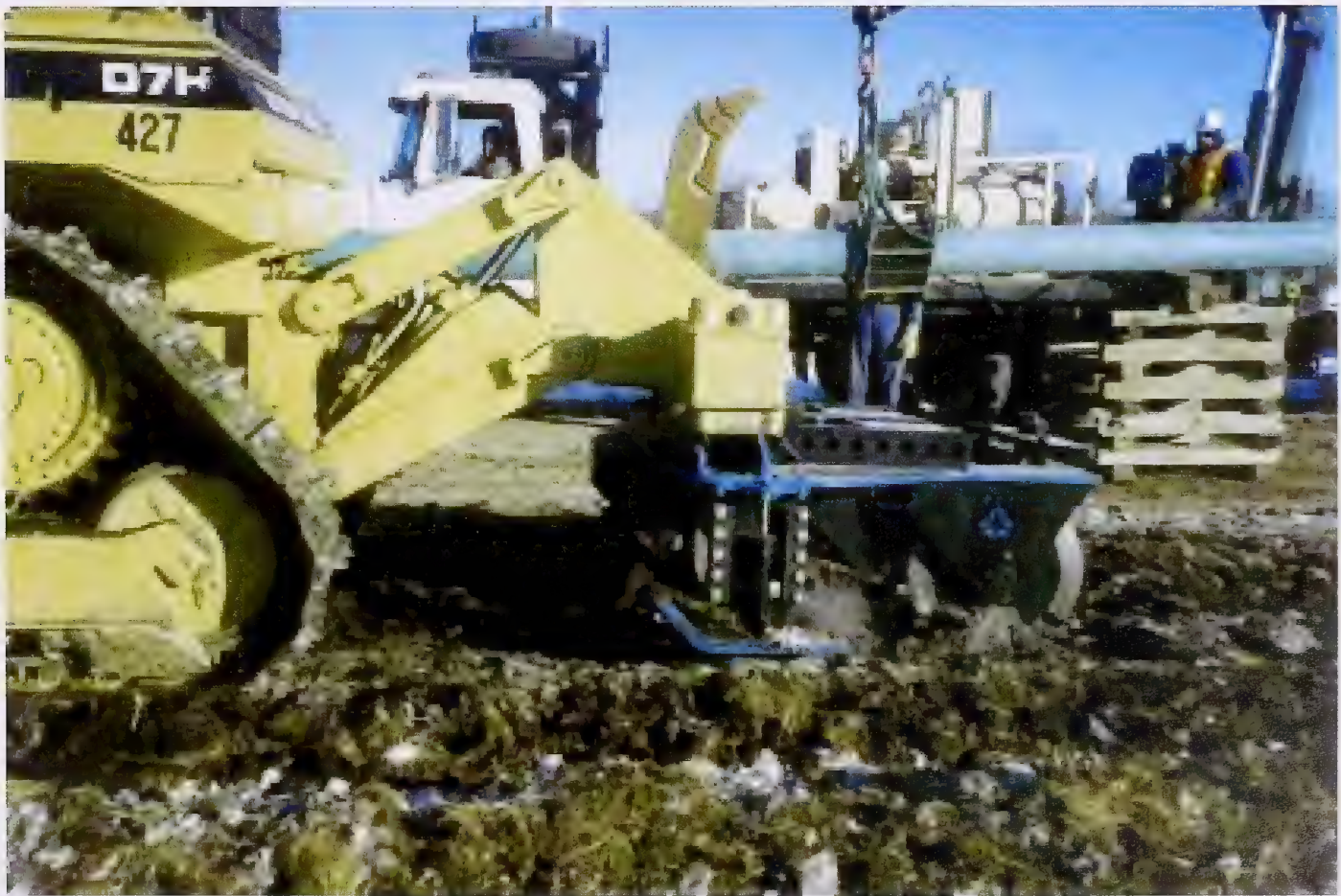
Photo 49 Frozen topsoil cutter mounted on a dozer.
